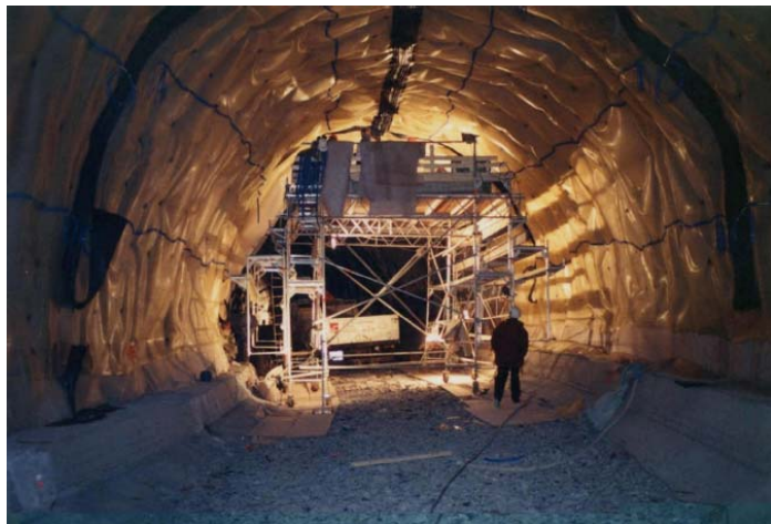
(Fig. 28) Geotextiles impermeable
